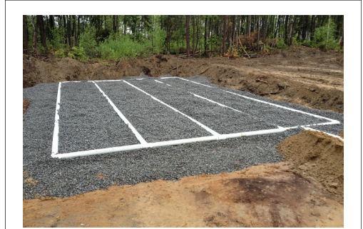
Fig. 3. Photo of a standard leaching bed before backfilling
